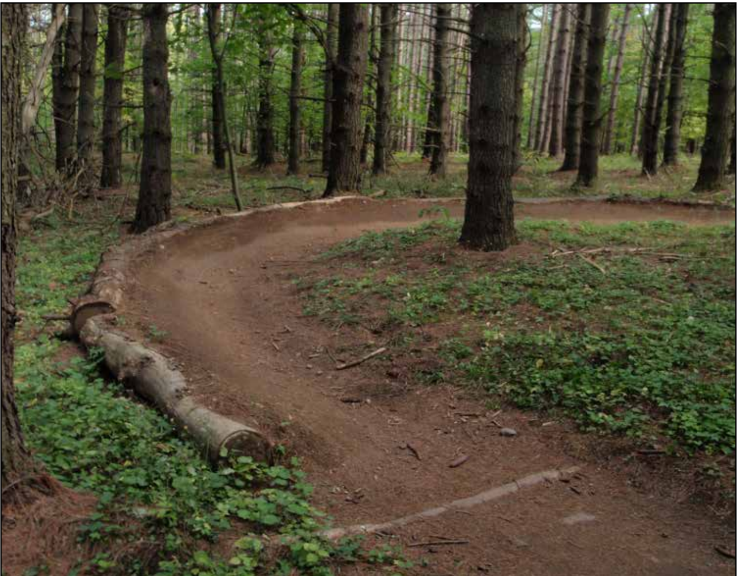
This picture shows an inslope turn in the Hardy Road mountain bike trail network. These trails features are only used on mountain bike trails and not on any other kind of trail on the Forest Preserve.
