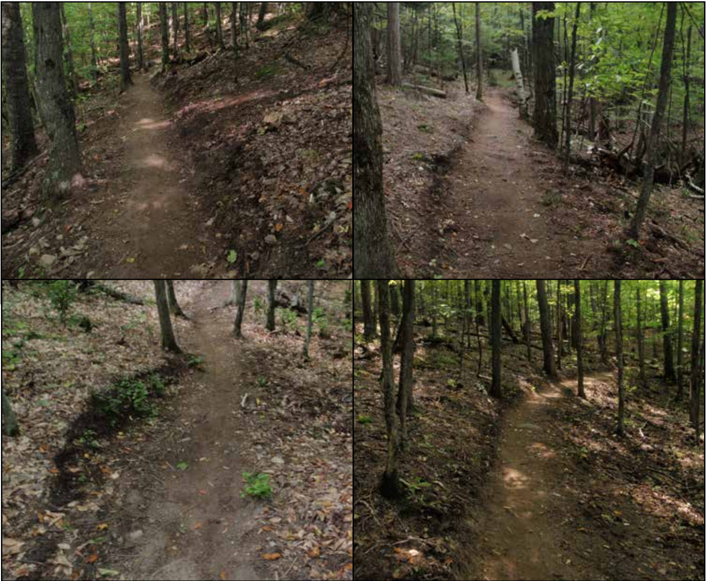
Pictures above show different bench cuts (“side slope management”) made in new sections of the Hardy Road mountain bike trails in the Wilmington Wild Forest area. Bench cuts are a frequently used technique in side slope management and, arguably more than any other trail design and construction technique, alters a trail area and changes the wild forest character of the Forest Preserve.
