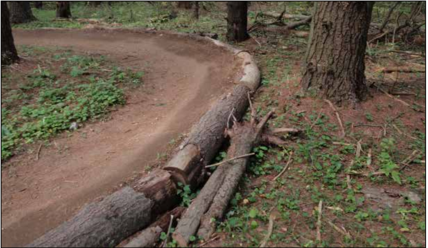
Picture above shows a specially built banked turn, known as an inslope corner, on a section of the Hardy Road mountain bike trail network in the Wilmington Wild Forest. It's hard to imagine a scenario where this trail is appropriate for shared "equestrian" uses (horse riding) and would not be damaged. This is also a feature not used on a foot trail.
