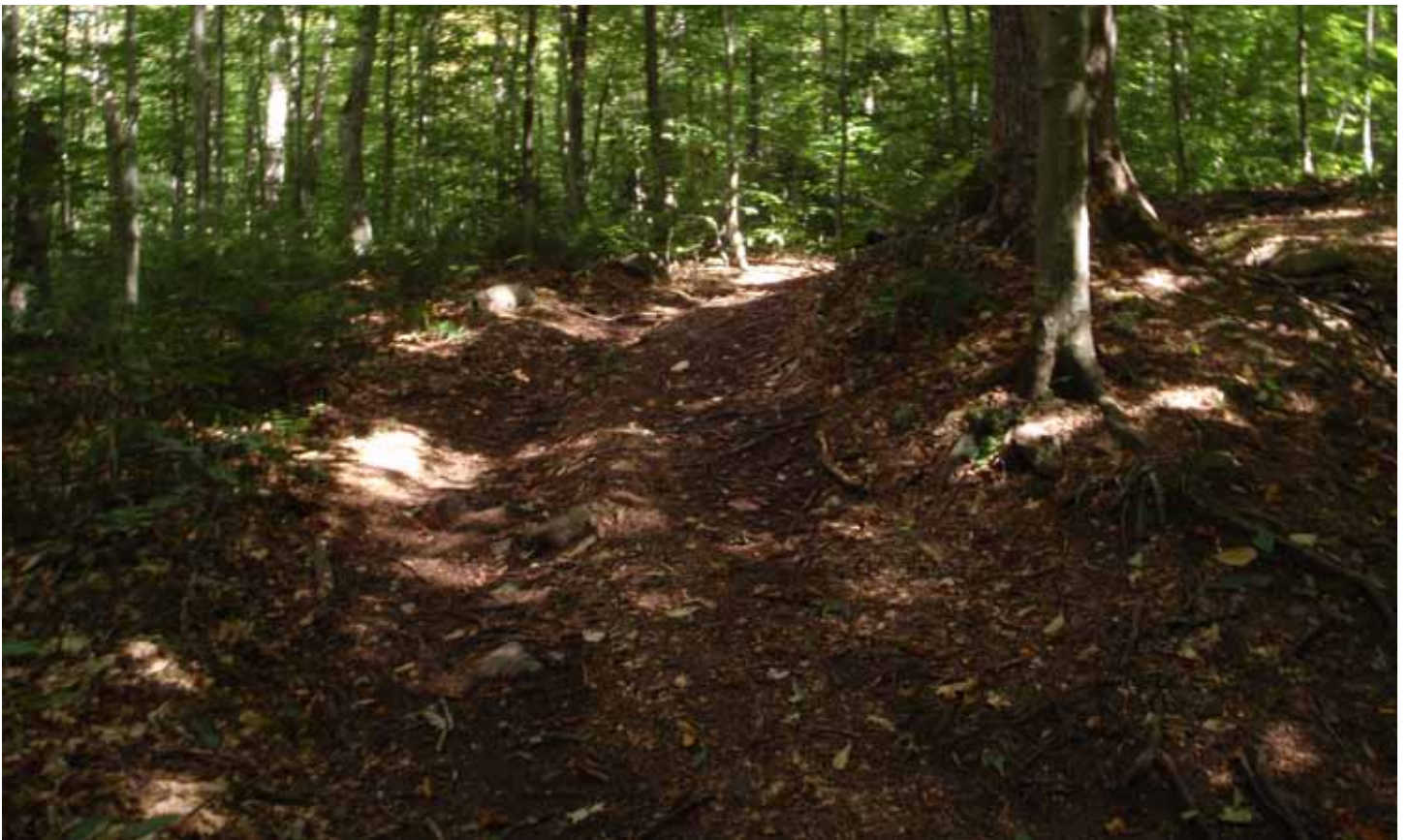
More pictures that show natural resource damage along the Gull Lake Trail in the Black River Wild Forest from illegal ATV use. This trail corridor has suffered extensive damage. Compacted soils have experienced considerable damage.
