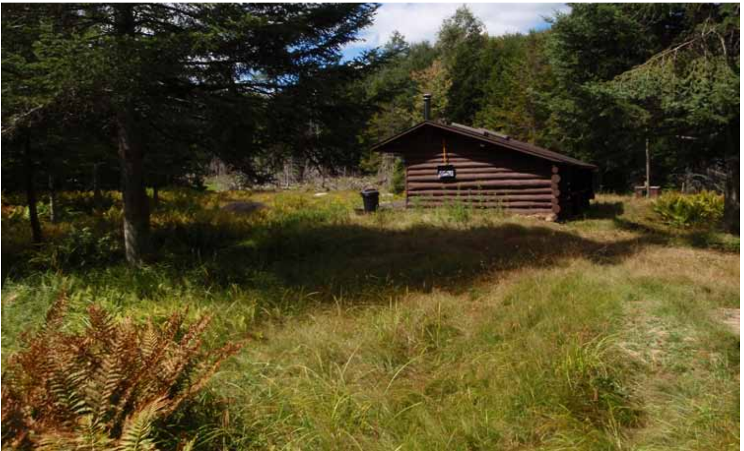
The Chub Pond Lean-to has seen a lot of clearing in the meadow around it. A lawn mower stored on site has prevented the forest from growing up around the lean-to. This is an abuse of the Forest Preserve.
