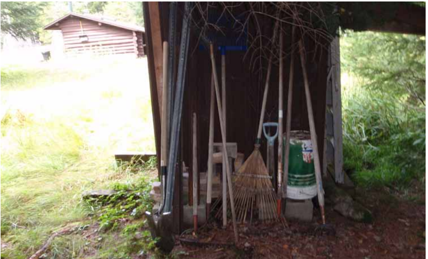
The Chub Pond Lean-to outhouse is being used as a storage shed to hold chemicals. Various yard tools are stored outside the outhouse.
