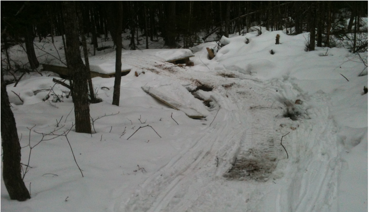
Incomplete bridge through what appears to be a class 1 wetland system. Snowmobiles are driving through the wetland, which has pooled water in places. No silt fences or mitigation was visible.
