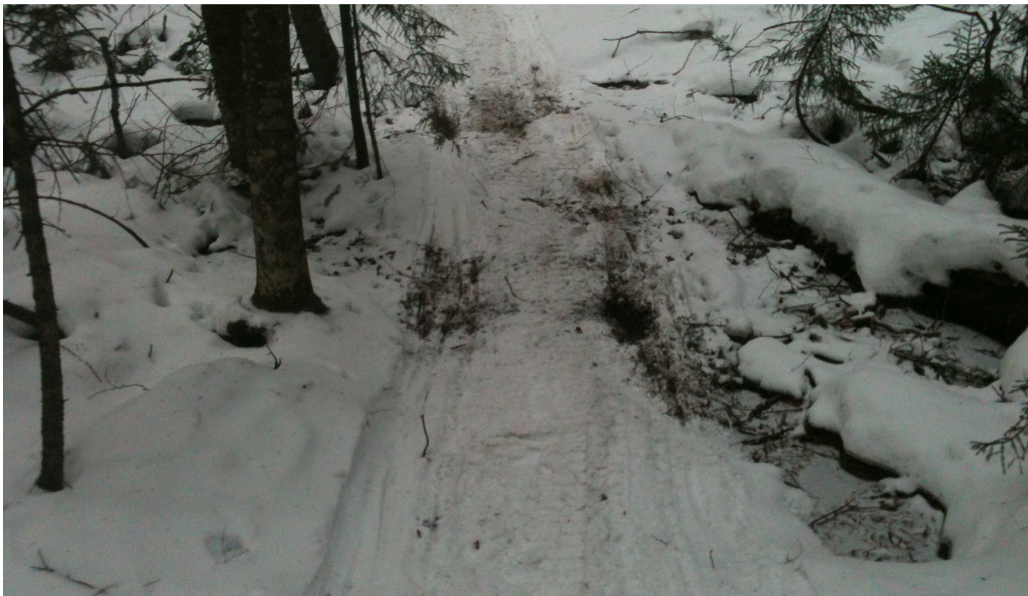
Another section of trail built through a wetland or stream crossing with no bridge or protection for the stream. Snowmobiles are driving through the stream channel.
