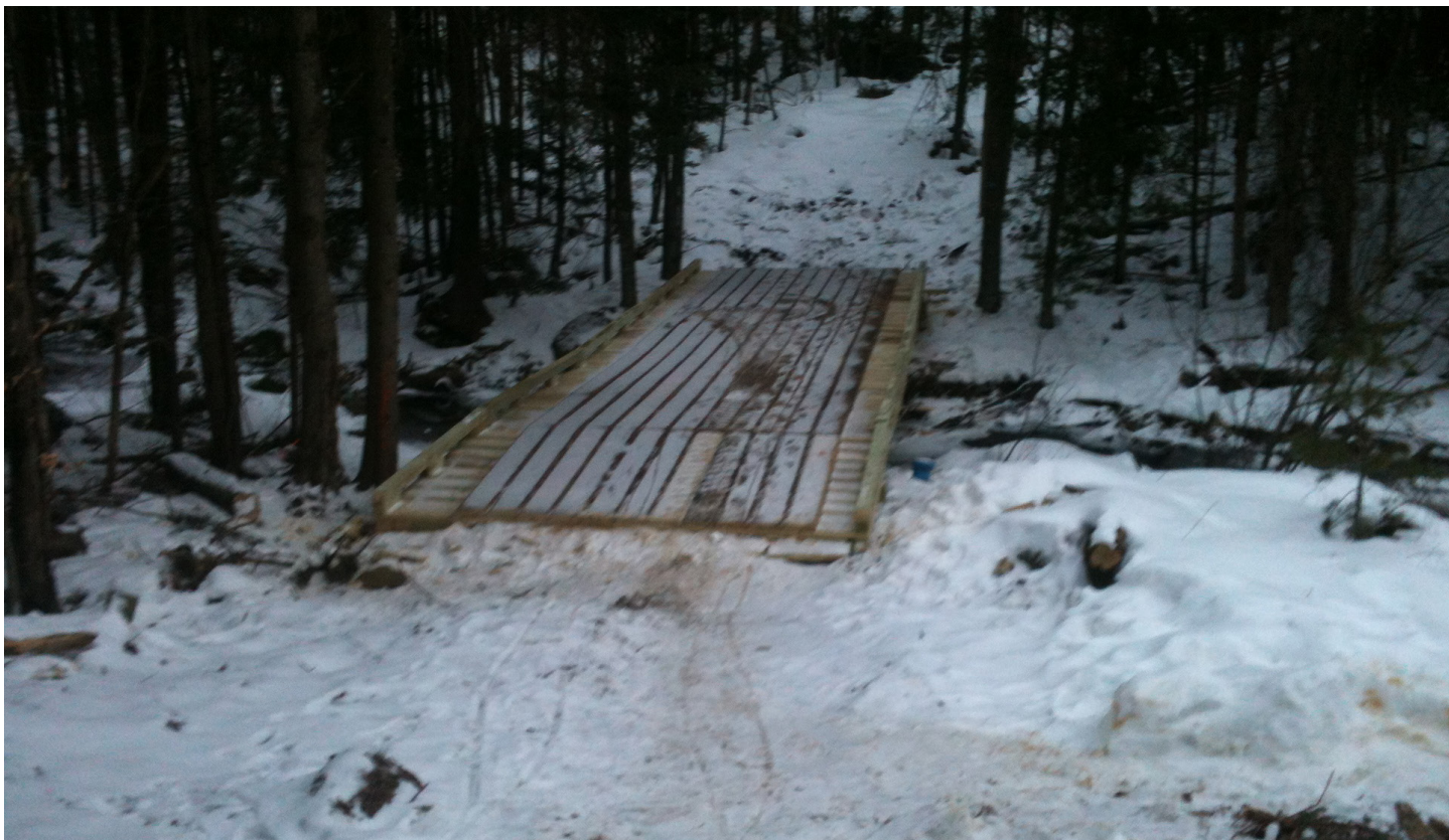
Extensive disturbed area, likely more than 1 acre, around the new bridge at the outlet of the Raquette Lake Reservoir. Lots of debris. No silt fences or mitigation was visible.
