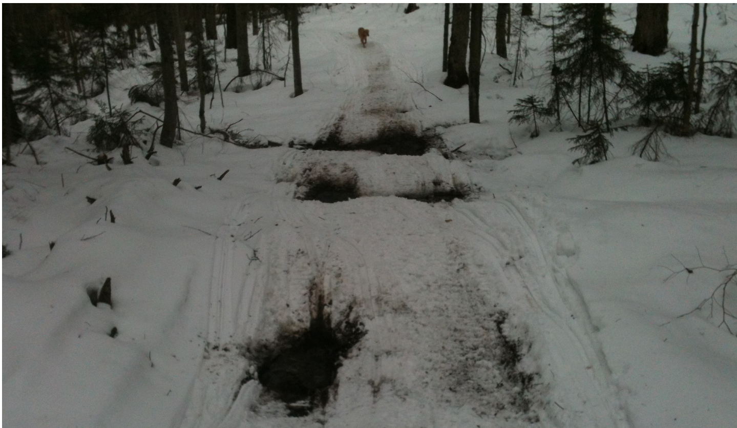
Part of trail where no bridge was built through a large wetland. Snowmobiles are driving through the wetland, which has pooled water in places.
