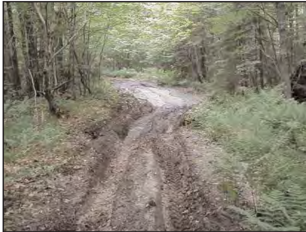
Top left: ATV damage ruts road in a wetland area on the Chubb Pond Trail. Right: Herkimer Landing Road. Bottom left: ATV damage on the Black Creek Lake Road. Middle: Damage from ATV trespass on the South Lake Trail. Right: ATV damage on the Bear Creek Road.
