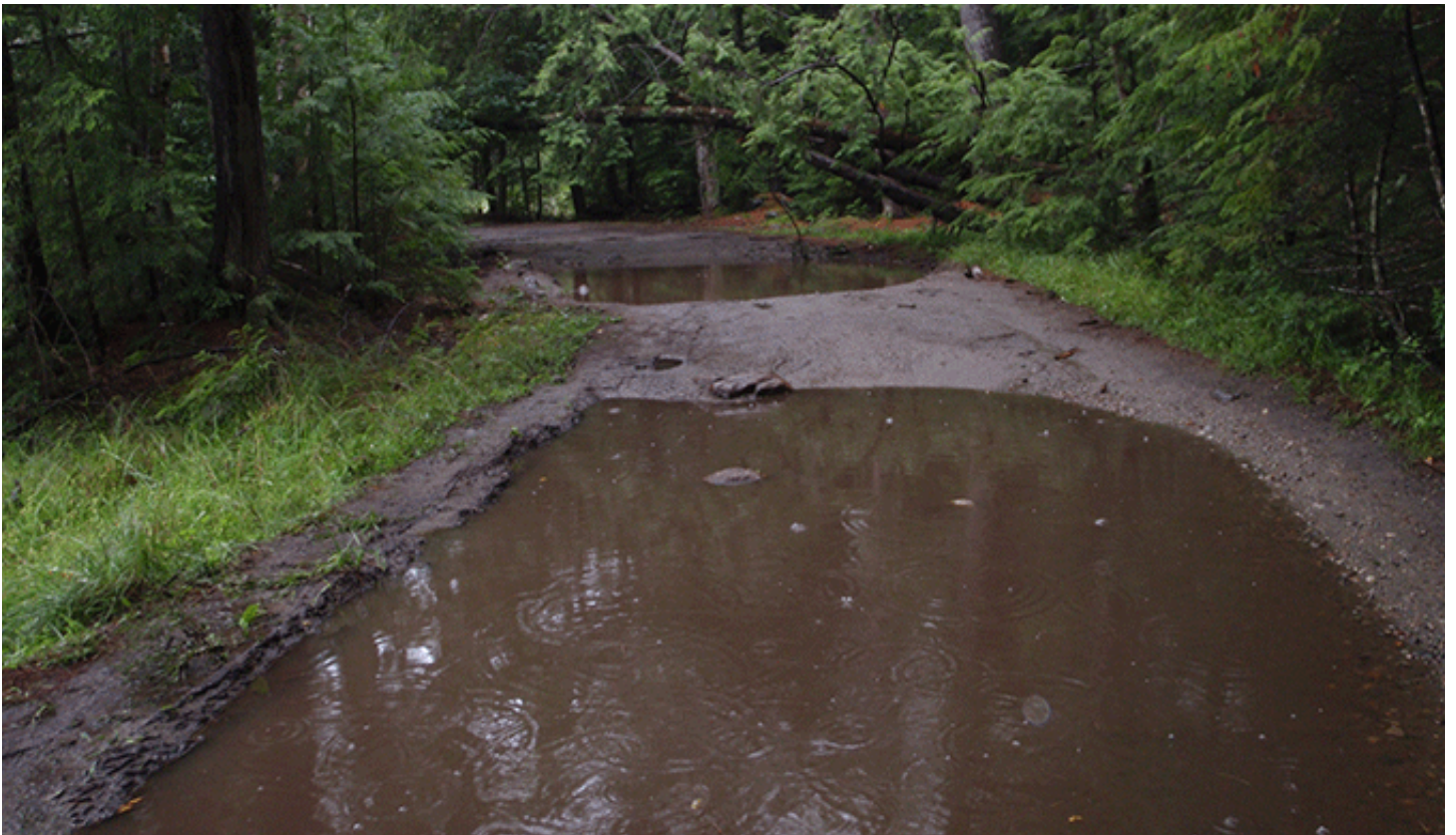
Two sections on the Crane Pond Road that show extensive drainage problems due to soil compaction and degradation from motorized uses.
