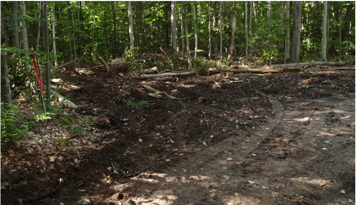
Two more pictures that show areas of the Bear Creek Road where DEC has undertaken work to clear the roadside and expand the width of the road. In many places the width of the Bear Creek Road corridor has been expanded 50% or more.
