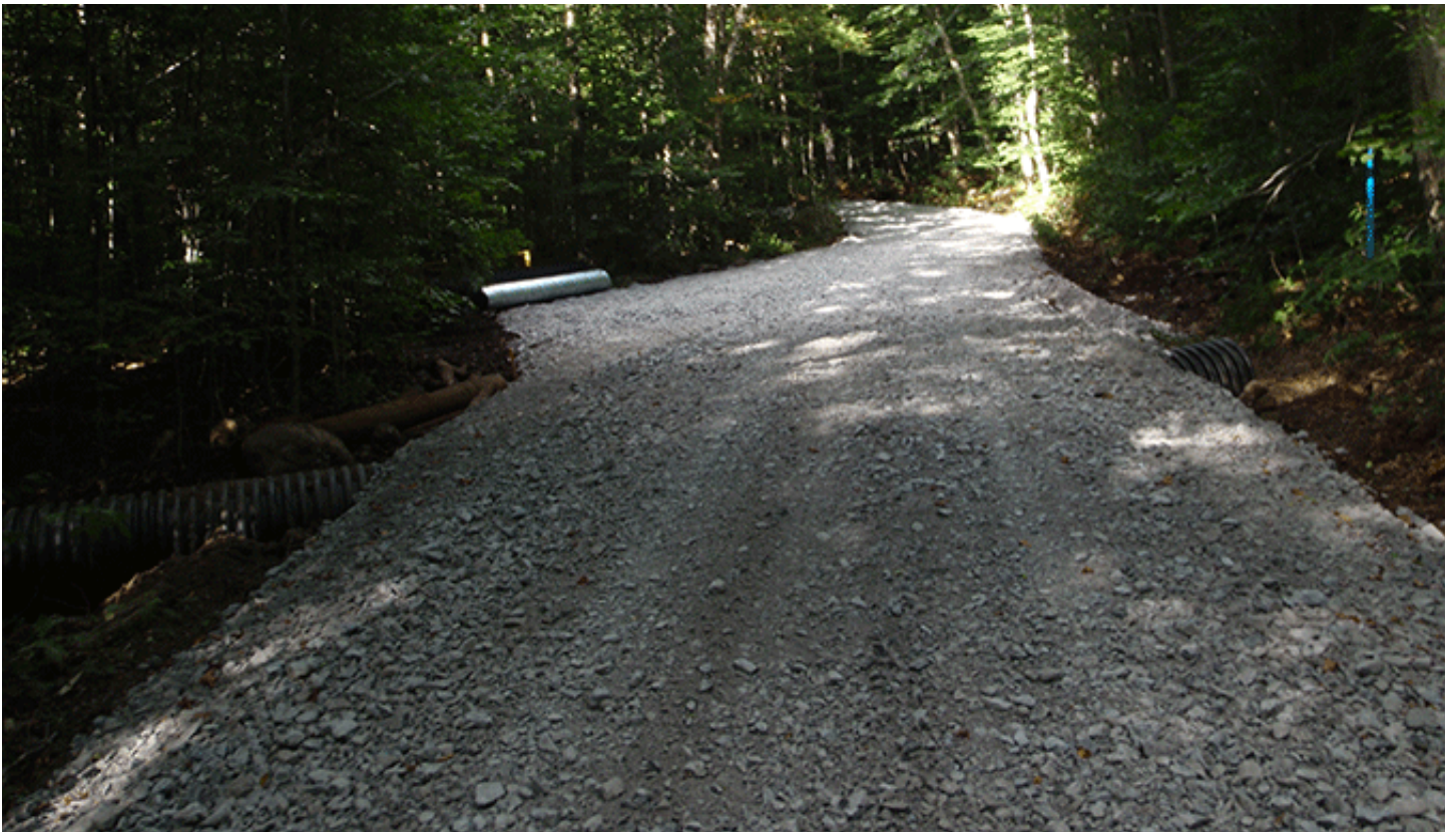
Two areas of the Bear Creek Road that have been reconstructed. The road has been widened with a deep gravel surface. Two small pull-offs are pictured on these stretches. Small and large pull-offs are a regular feature on this road.
