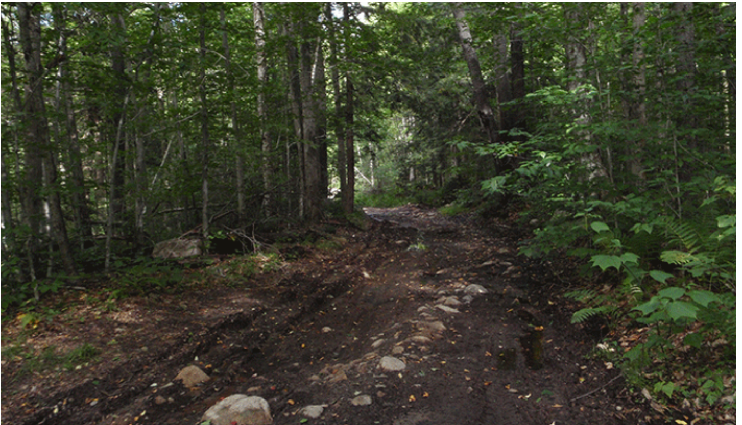
Two pictures of the current condition of the Bear Creek Road in the Black River Wild Forest area. Though heavily rutted by legal and illegal motor vehicle use, especially by ATVs, the road corridor is narrow in most places and is 9-11 feet in width.
