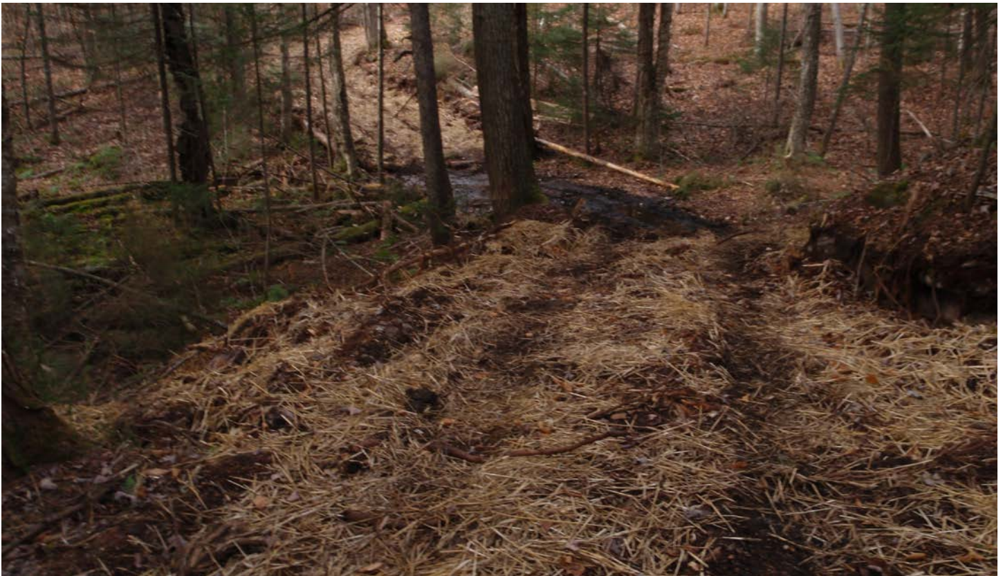
Two more pictures of the construction of the class II community connector snowmobile trail around Harris Lake. These pictures show areas far in excess of the 12 foot maximum width for slopes or curves and 9 feet for straight areas. This excessive widening of the trail surface causes unnecessary natural resource damage to the Forest Preserve.
