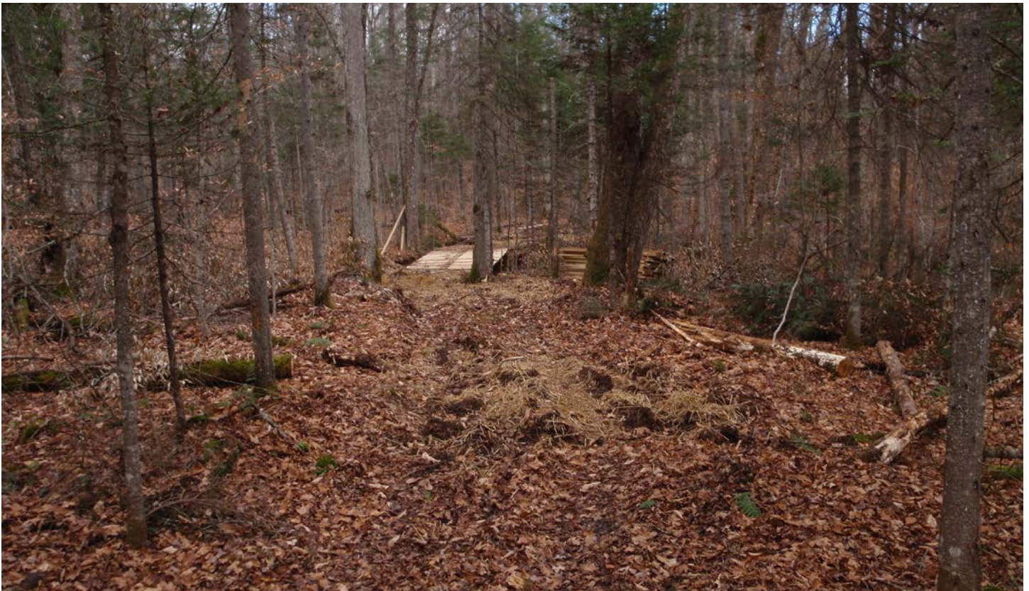
Two more pictures of the construction of the class II community connector snowmobile trail around Harris Lake. These pictures show areas far in excess of the 12 foot maximum width for slopes or curves and 9 feet for straight areas. This excessive widening of the trail surface causes unnecessary natural resource damage to the Forest Preserve. The bridge in the distance is 12.5 feet wide for reference.
