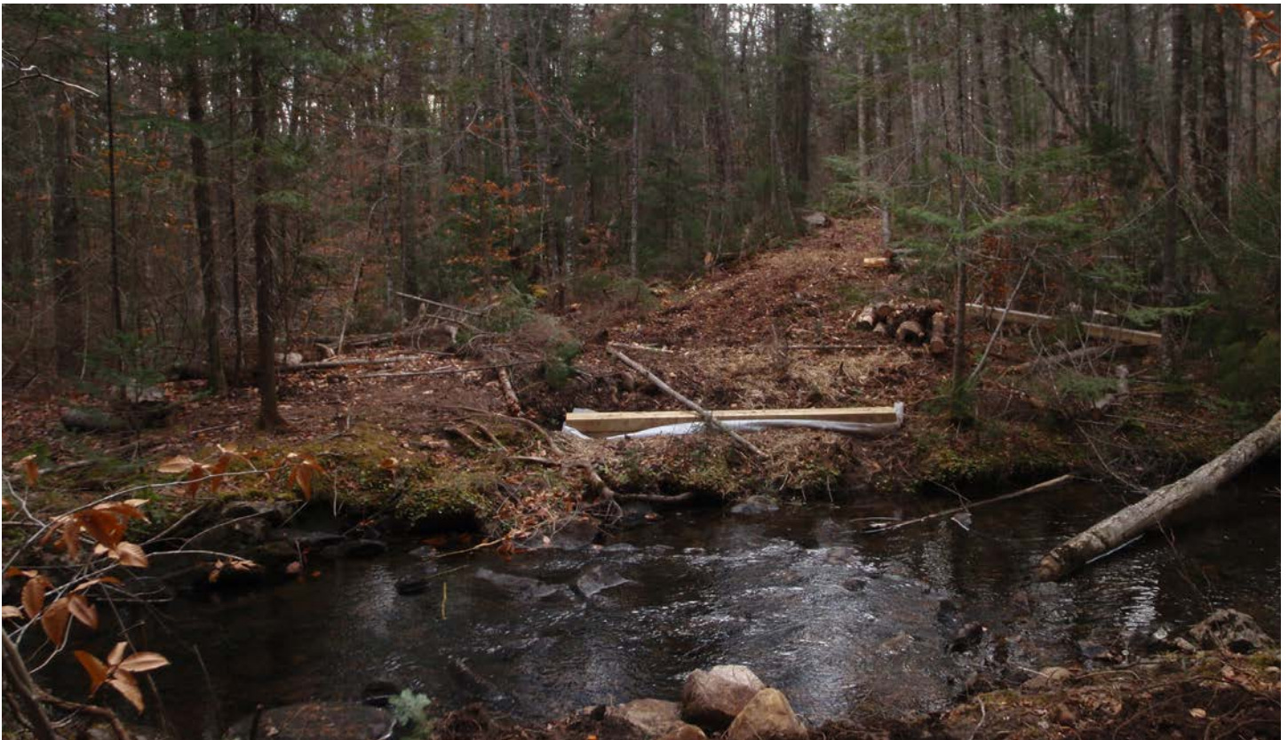
Two pictures that show bridge construction on the Harris Lake trail over a permanent stream. Though the DEC issued itself a Stormwater Management Permit for this project it failed to use any type of silt fencing and has exposed earth that runs right to the stream. This is not acceptable natural resource protection.
