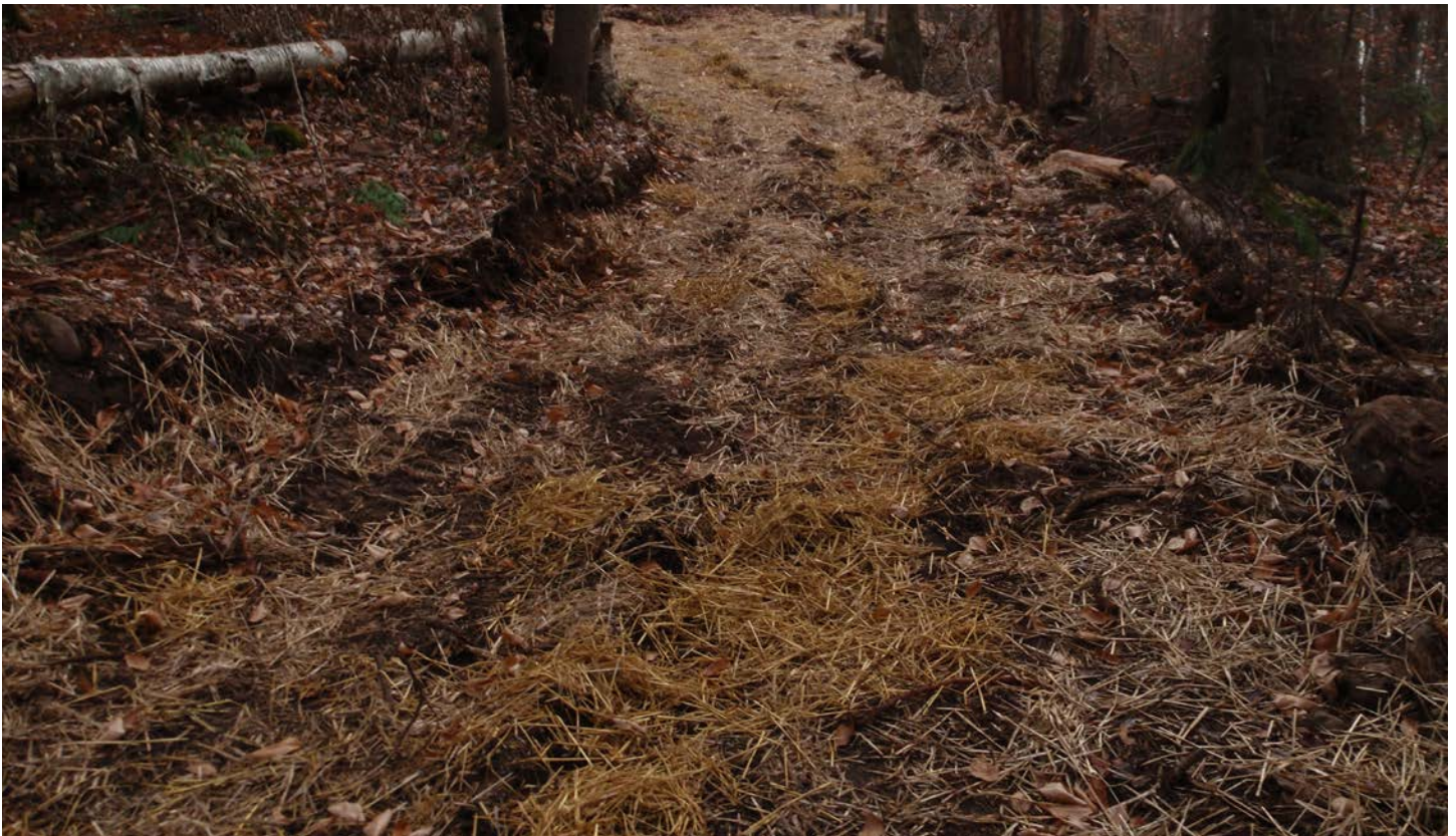
These pictures show extensive grading and levelling work on the Harris Lake trail. After extensive tree cutting, rock removal, filling in of hummocks, and complete destruction of the forest understory, grading and levelling dramatically change a trail.
