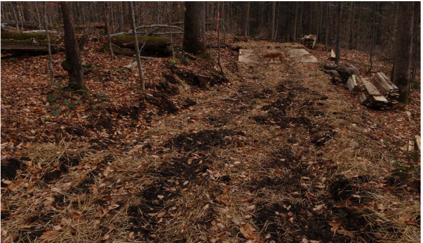
Two more pictures of the construction of the class II community connector snowmobile trail around Harris Lake. These pictures show areas far in excess of the 12 foot maximum width for slopes or curves and 9 feet for straight areas. This excessive widening of the trail surface causes unnecessary natural resource damage to the Forest Preserve. The bridge in the bottom picture is 12.5 feet wide for reference.
