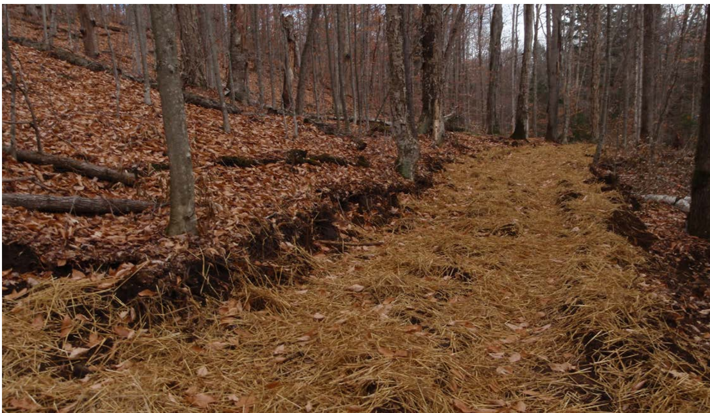
These pictures show extensive grading and “bench cutting” on the Harris Lake trail. After extensive tree cutting, rock removal, filling in of hummocks, and complete destruction of the forest understory, grading and bench cutting dramatically change a trail.
