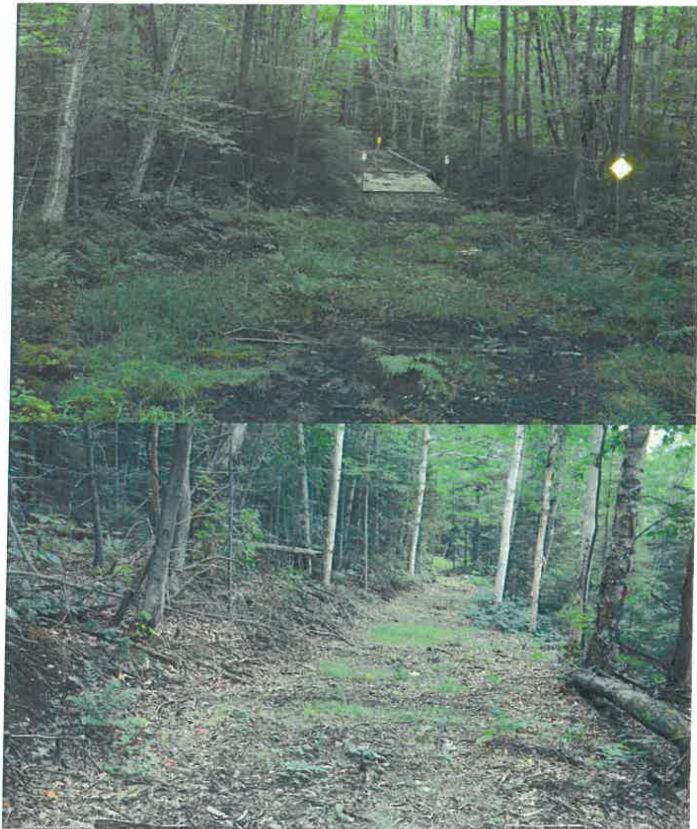
The pictures above show the widths of class II community connector snowmobile trails. The top picture shows a 12-foot-wide bridge. The area in front of the bridge is clearly much wider. The lower picture shows a typical stretch of connector trail with cleared bench cuts and a wide cleared trail surface area.
