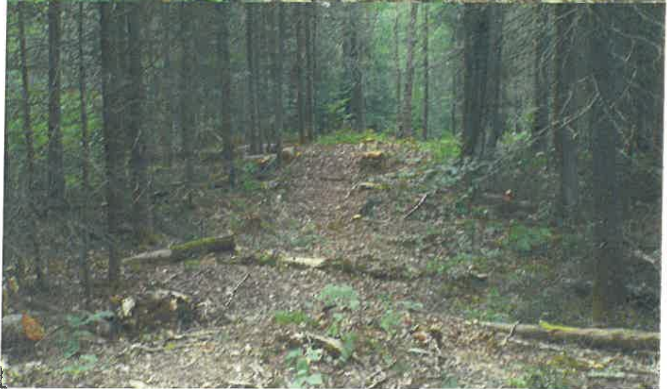
The pictures above show sections of new class II community connector snowmobile trails. These wide trails require significant tree cutting. Tree stumps will be prominent on these trails for years to come.
