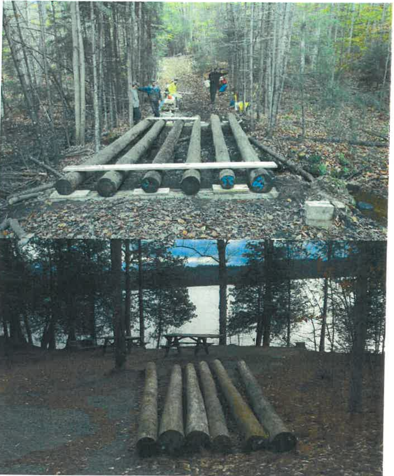
The pictures above show large poles, chemically treated and imported from outside of the area, used as structural beams for 12-foot-wide class II community connector trail bridges in the Moose River Plains and other areas.
