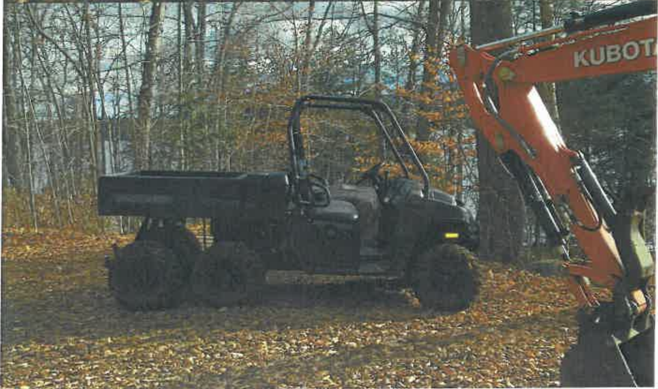
The pictures above show the heavy machinery used by the DEC to build new class II community connector snowmobile trails. Foot trails are built with hand tools.
