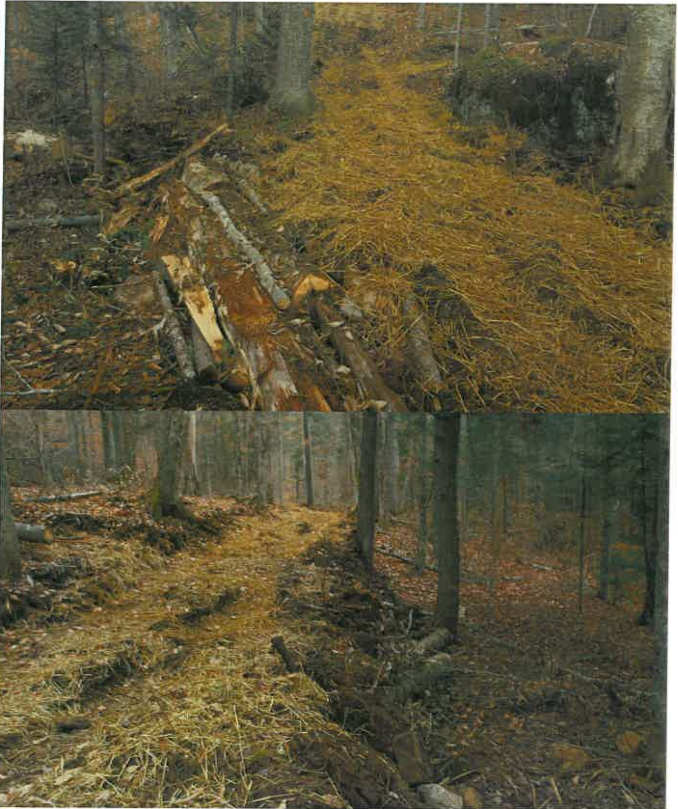
The pictures above show trailside debris used to build up the downslope side of class II community connector snowmobile trails. This type of activity is not undertaken on foot trails.
