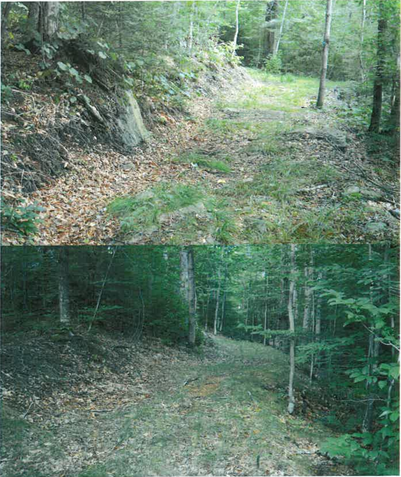
The pictures above were taken in the summer of 2016 on the Seventh Lake Mountain Trail, a newly constructed class II community connector snowmobile trail located in the Moose River Plains Wild Forest area, part of the Adirondack Forest Preserve. These pictures show visible man-made bench cuts that have not revegetated.
