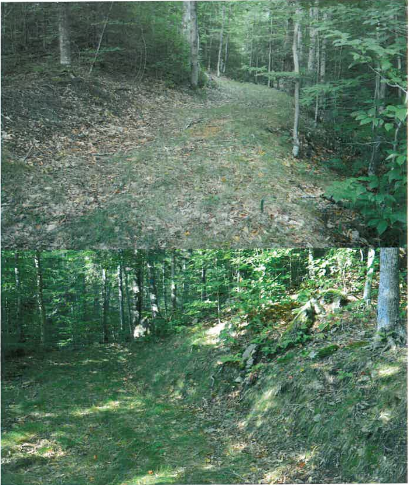
The pictures above were taken in the summer of 2016 on the Seventh Lake Mountain Trail, a newly constructed class II community connector snowmobile trail located in the Moose River Plains Wild Forest area, part of the Adirondack Forest Preserve. These pictures show visible man-made bench cuts widely used on this trail.
