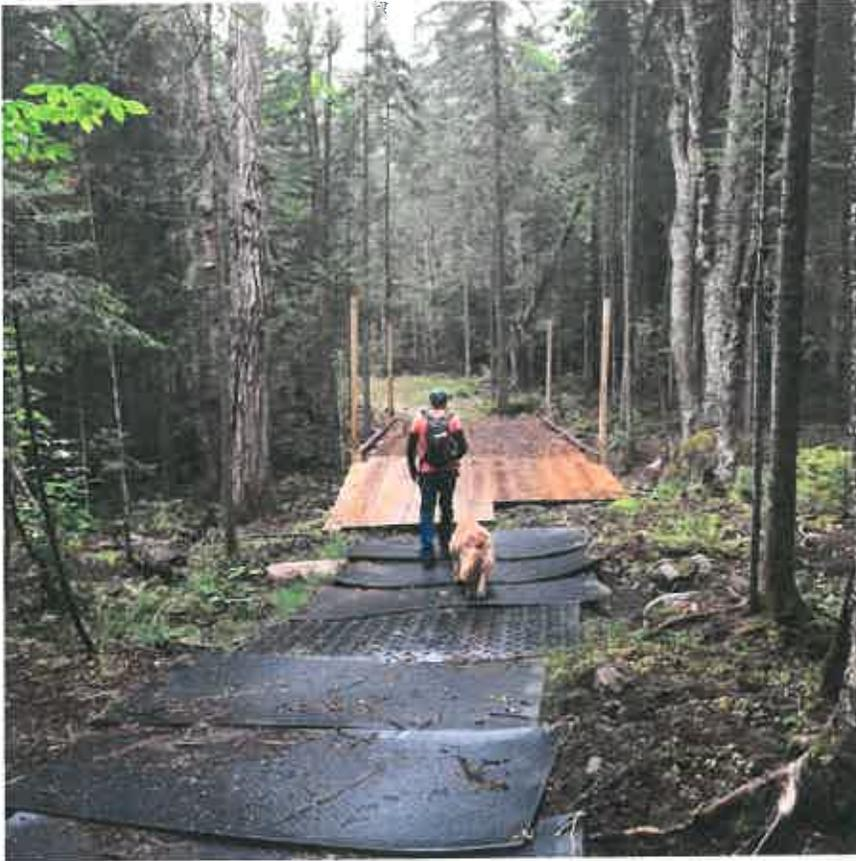
**Photo 7: Sturdy 12' wide wooden bridge installed along snowmobile route, with 4 corner posts to signal bridge location during deep snow conditions. The bridges were constructed of several layers of 2" thick treated lumber, mounted on what appeared to be treated utility poles for structural support.**
