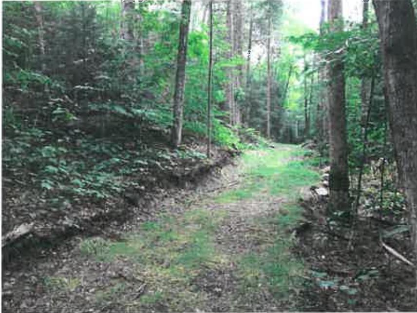
**Photo 2:** Road-like character of snowmobile trail. Also visible in this photo are "bench cuts" where soil was cut away from the slope to build the trail.
