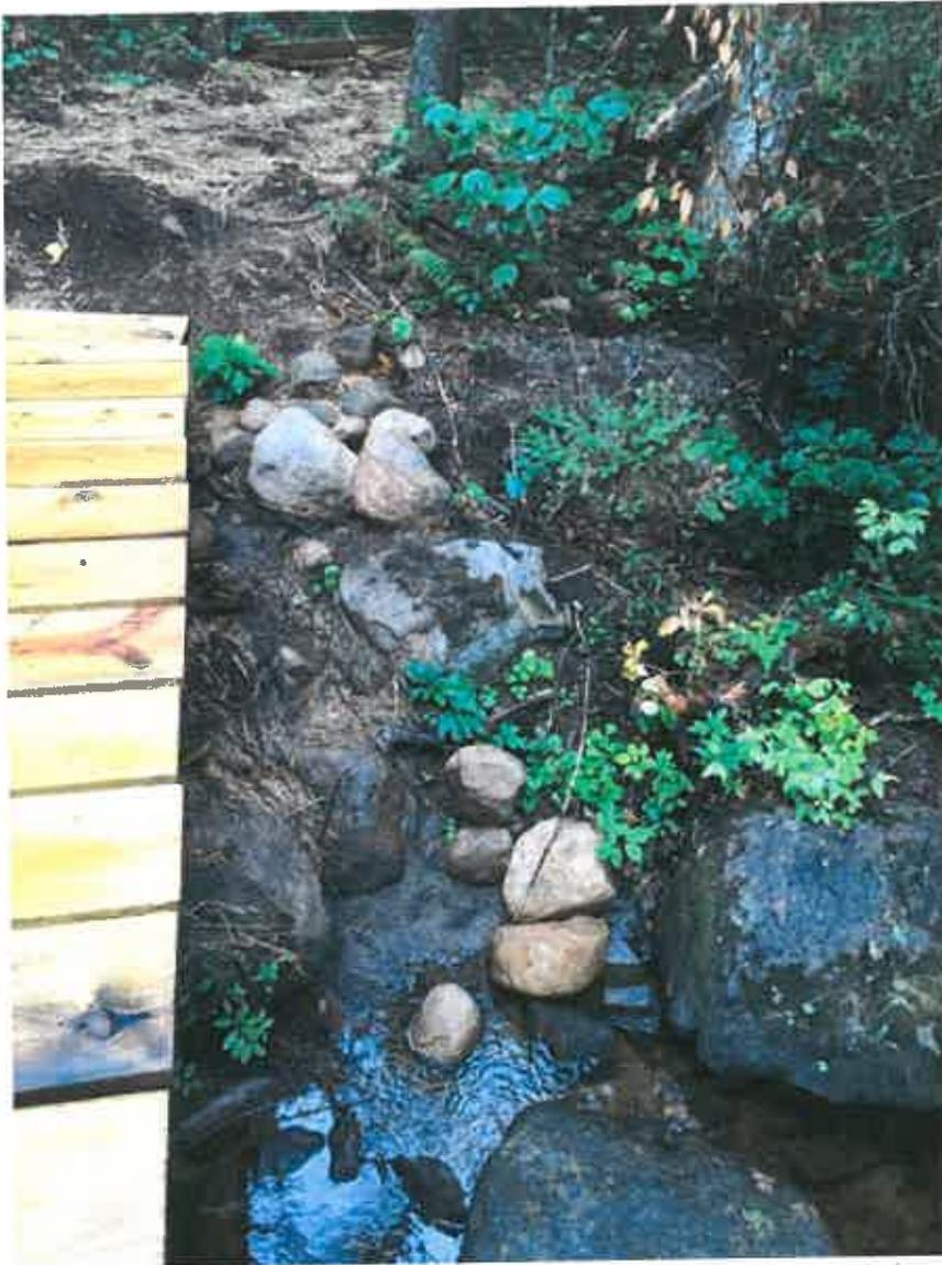
Photo 30: Soil erosion along the edge of where a snowmobile trail bridge adjoins the stream bank.
