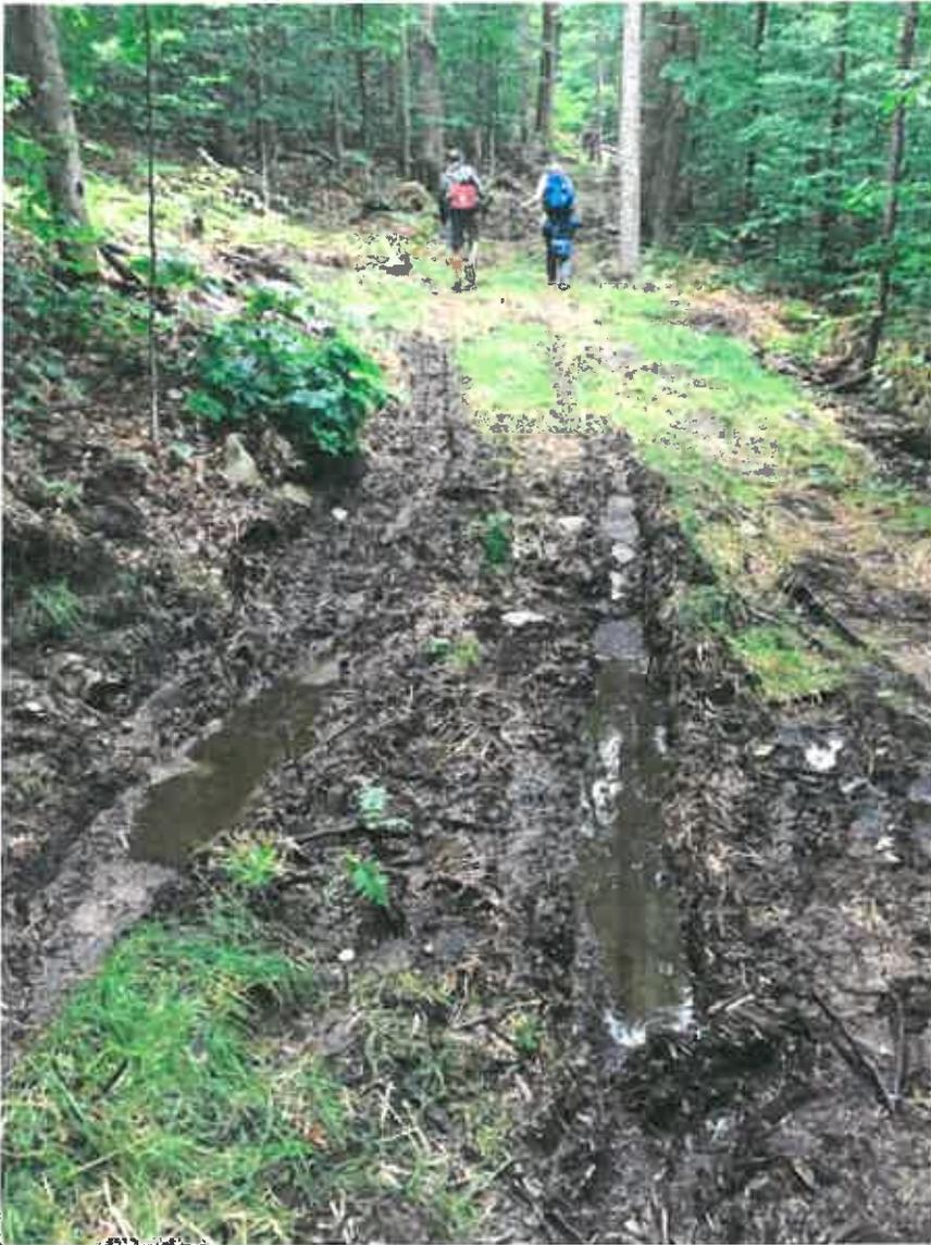
**Photo 11: Section of snowmobile trail passing through wet soil conditions, leading to muddy ruts and standing water.**
