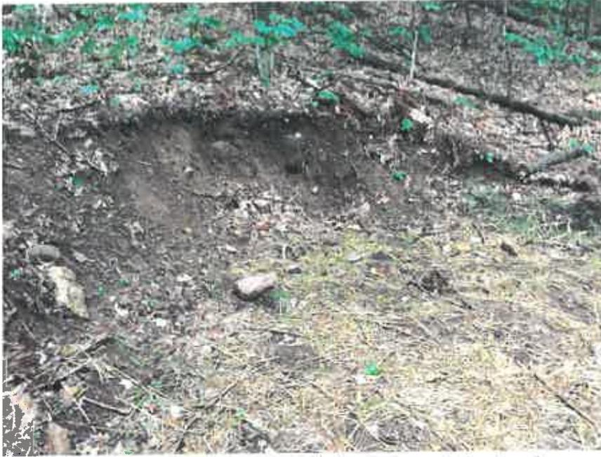
**Photo 27: An eroding "bench cut" that occurred during the process of constructing a snowmobile trail.**
