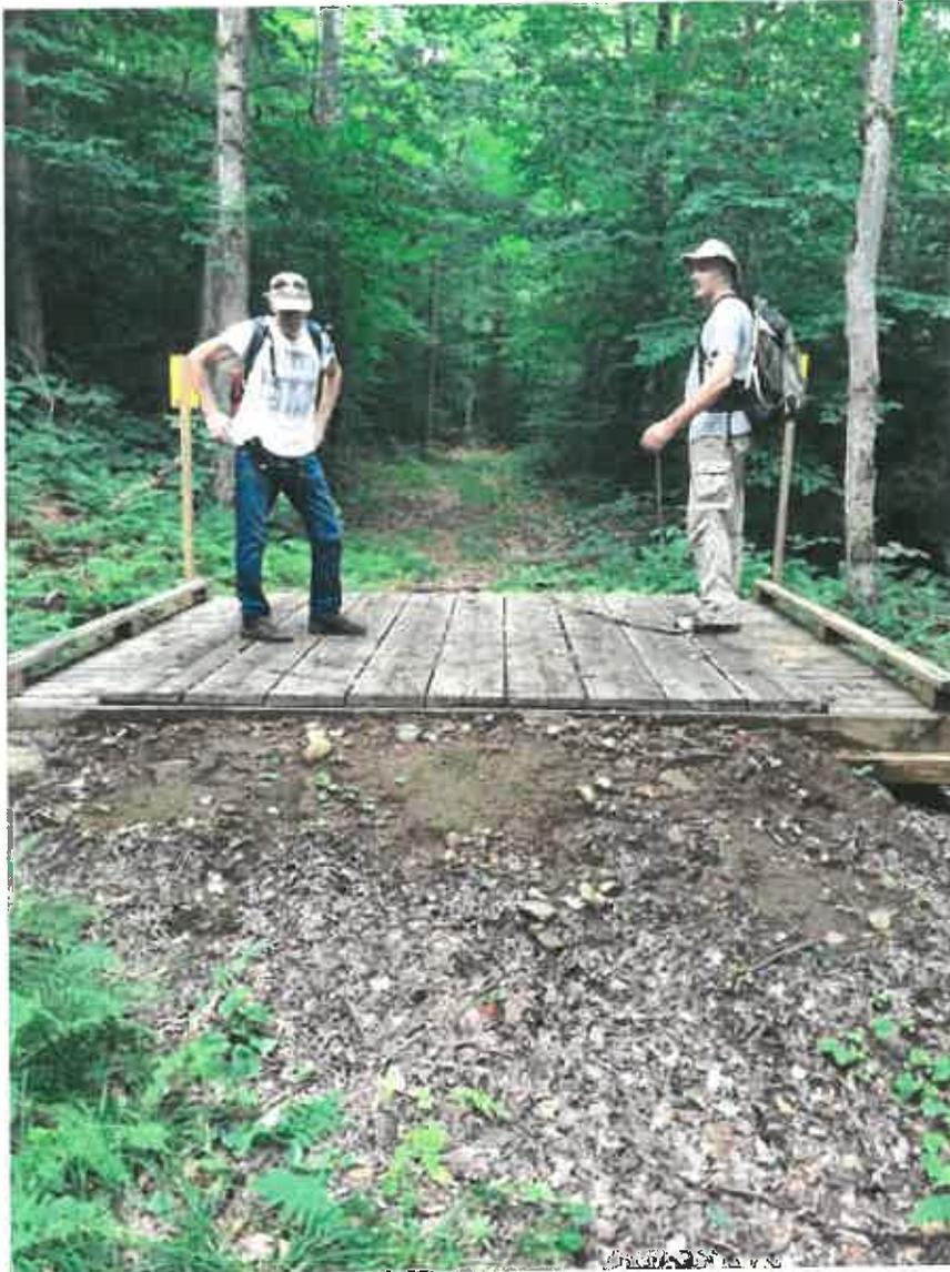
**Photo 29: Soil ramped up to the edge of a bridge along a snowmobile trail, creating the potential for erosion and sediment pollution in the adjacent creek.**
