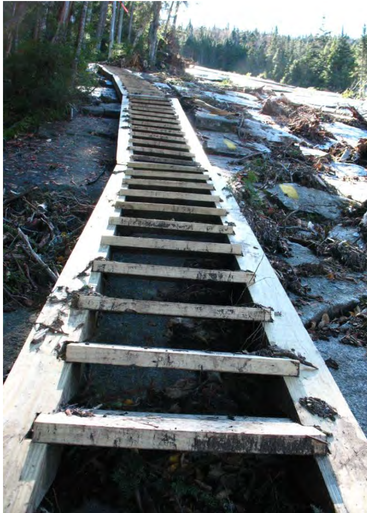
Picture of Ladders on Orebed Trail to Gothics Mtn, High Peaks Wilderness Area. Ladders are bolted to the bedrock to allow hikers to climb up the bedrock
