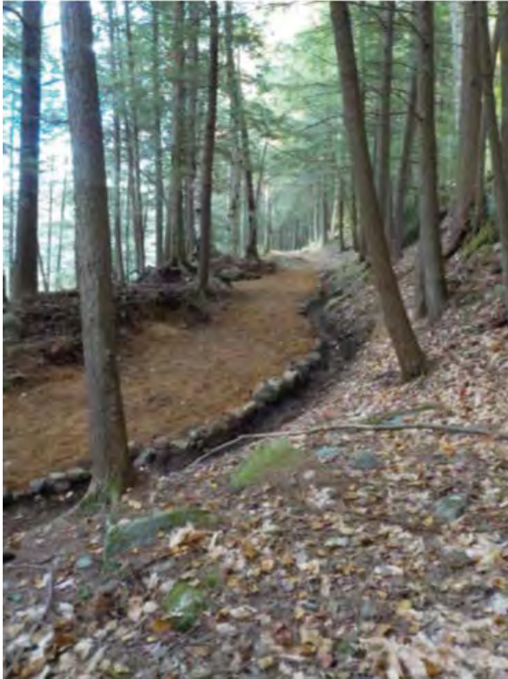
Picture of Turnpiking and linear drainage ditch on Pharaoh Lake Trail, Pharaoh Lake Wilderness Area Trail tread was raised so that water wasn't running down the middle of the trail.
