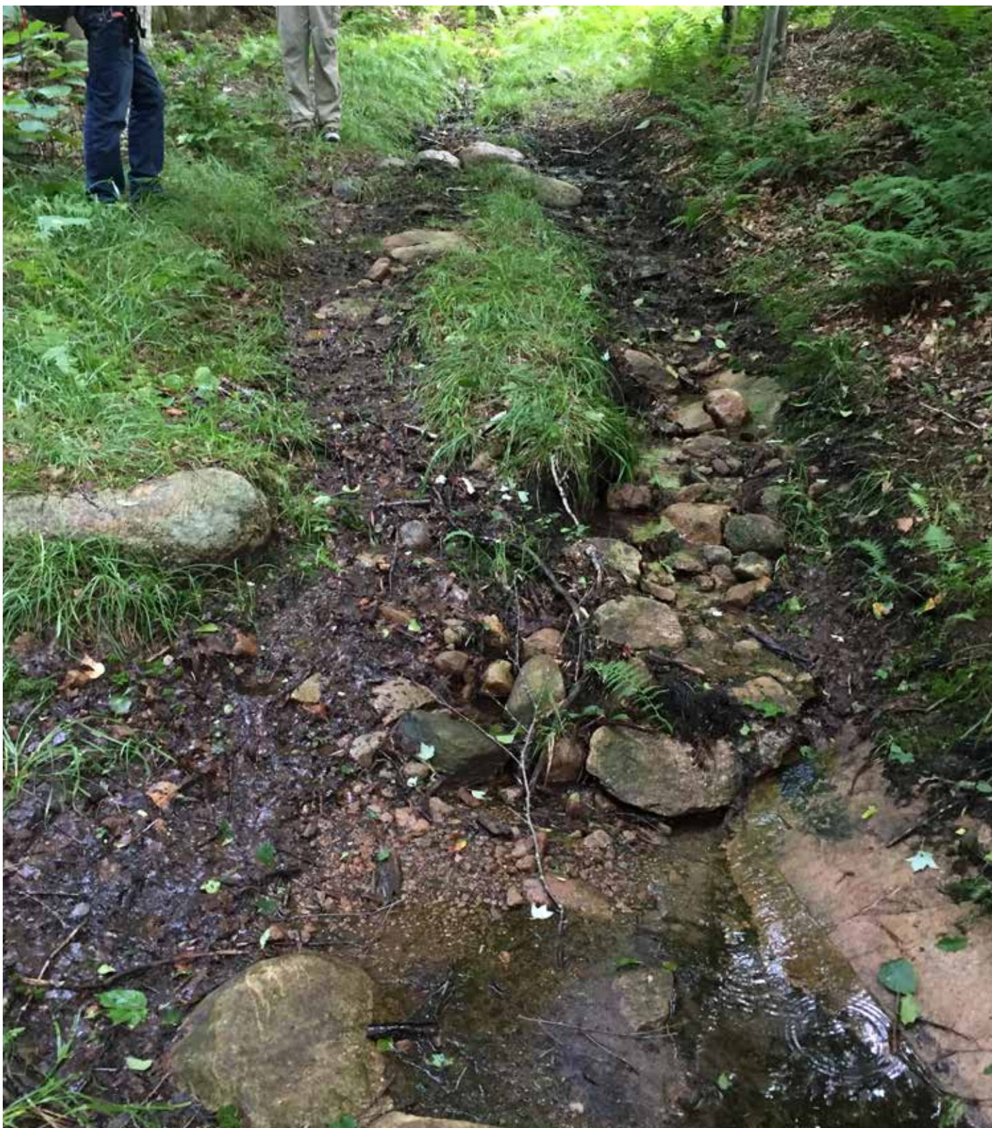
Community connector class II trails see dramatic removal of top soil and forest understory and as a result they are prone to erosion. This is a section word to bedrock on the Seventh Lake Mountain Trail in the Moose River Plains.
