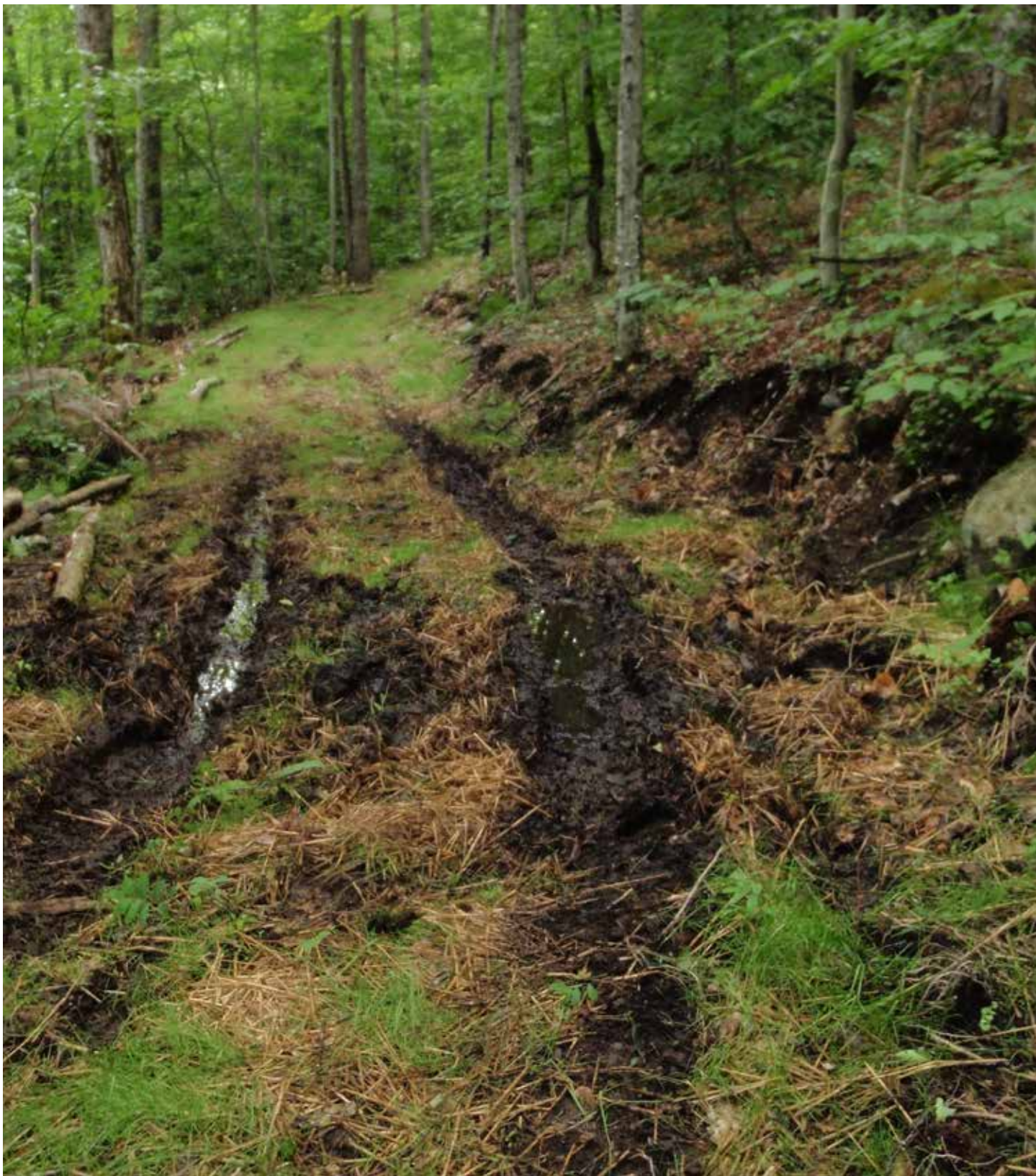
Another example of the damage to a forest caused by construction of a wide community connector class II trails. Here, benchcutting has been significant and the trail has been replanted with grass.
