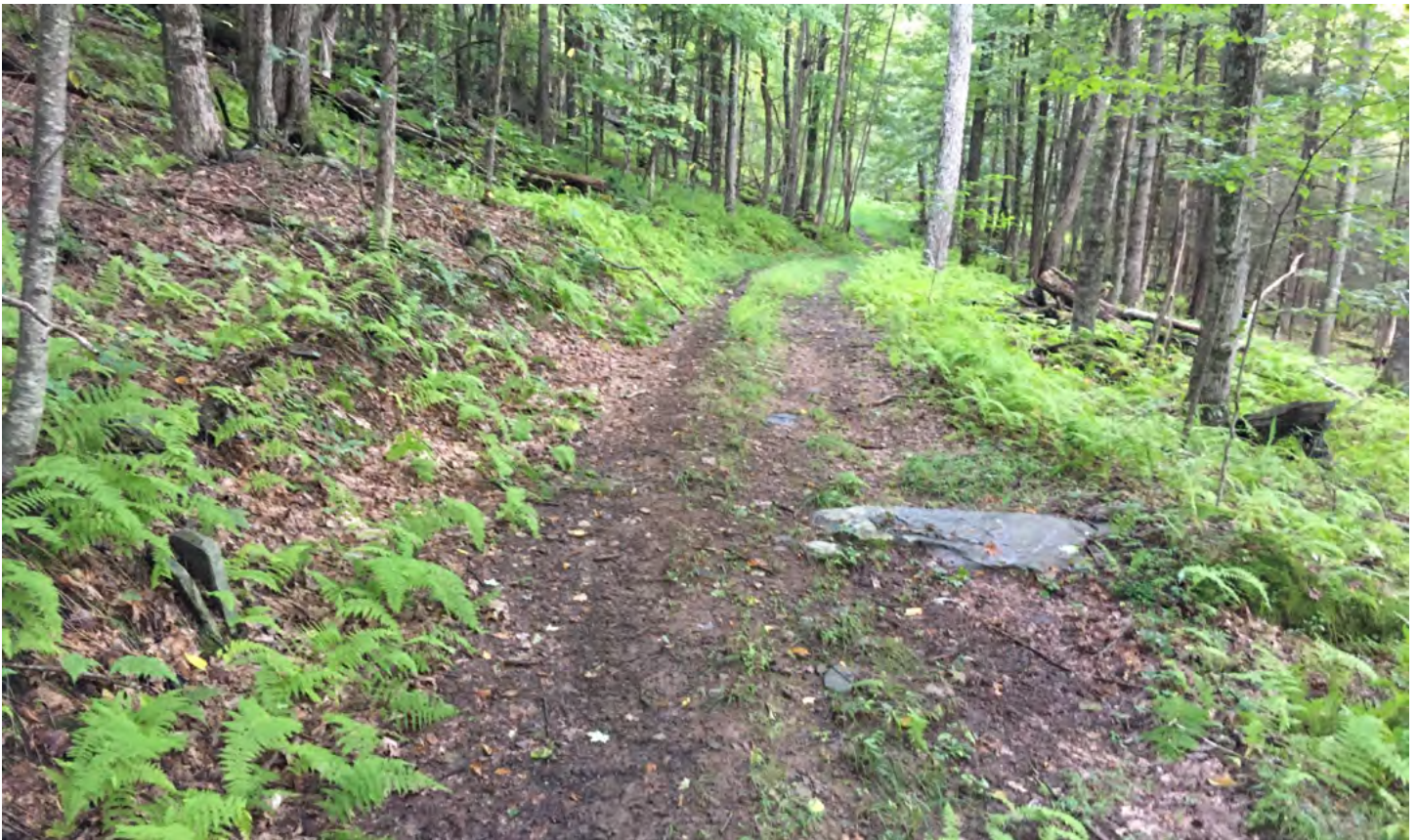
Two pictures of long benchcuts on the new multi-use trail in the Vernooy Kill State Forest. These pictures show two stretches of the trail with a long benchcut and flattened and graded surface. These sections are 12 and 13 feet wide of disturbed area respectively. They should have been no more than 6 feet wide.
