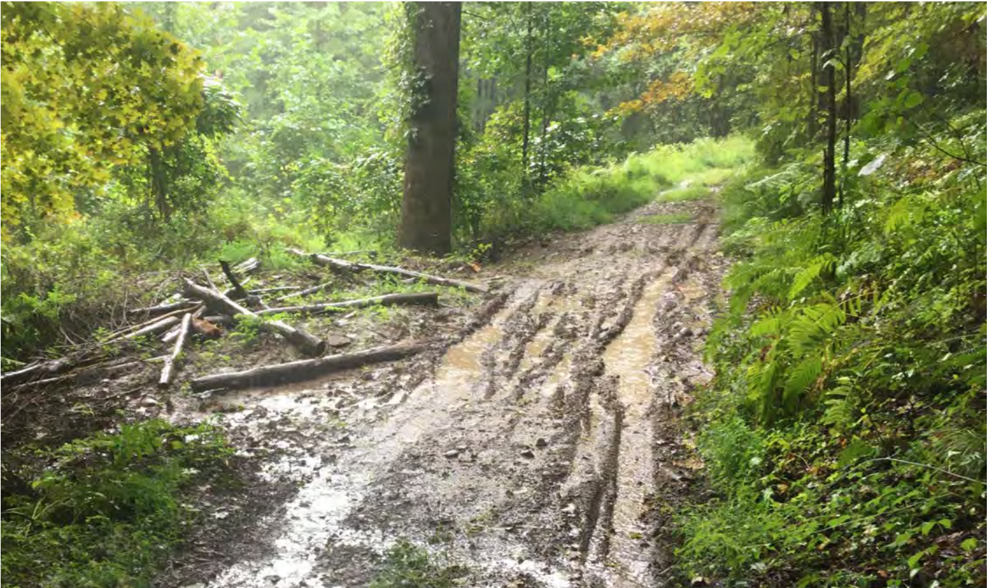
Three pictures of sections of the new multi-use trail in the Vernooy Kill State Forest. The two top pictures show rutted sections that are wide with extensive benchcuts. Bottom picture shows a wide section with a debris pile.
