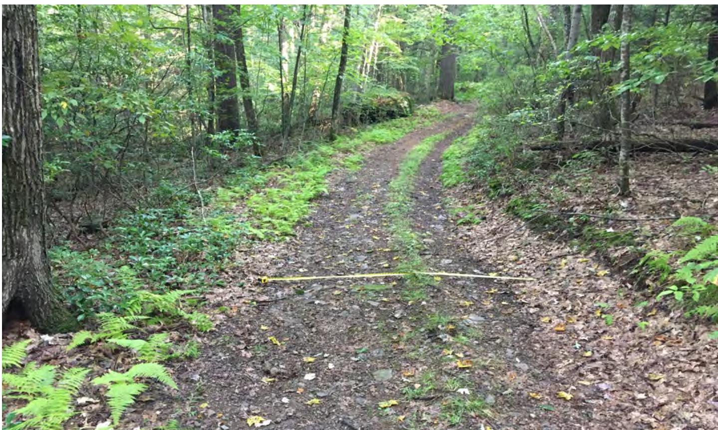
Two pictures of a typical scene from the new multi-use trail in the Vernooy Kill State Forest. The top shows a measuring tape at six feet on the trail tread. The bottom picture shows a measuring tape at 8 feet. The span of the disturbed area from the benchcut and grading is over 11 feet wide. The trail should be no more than 6 feet wide.
