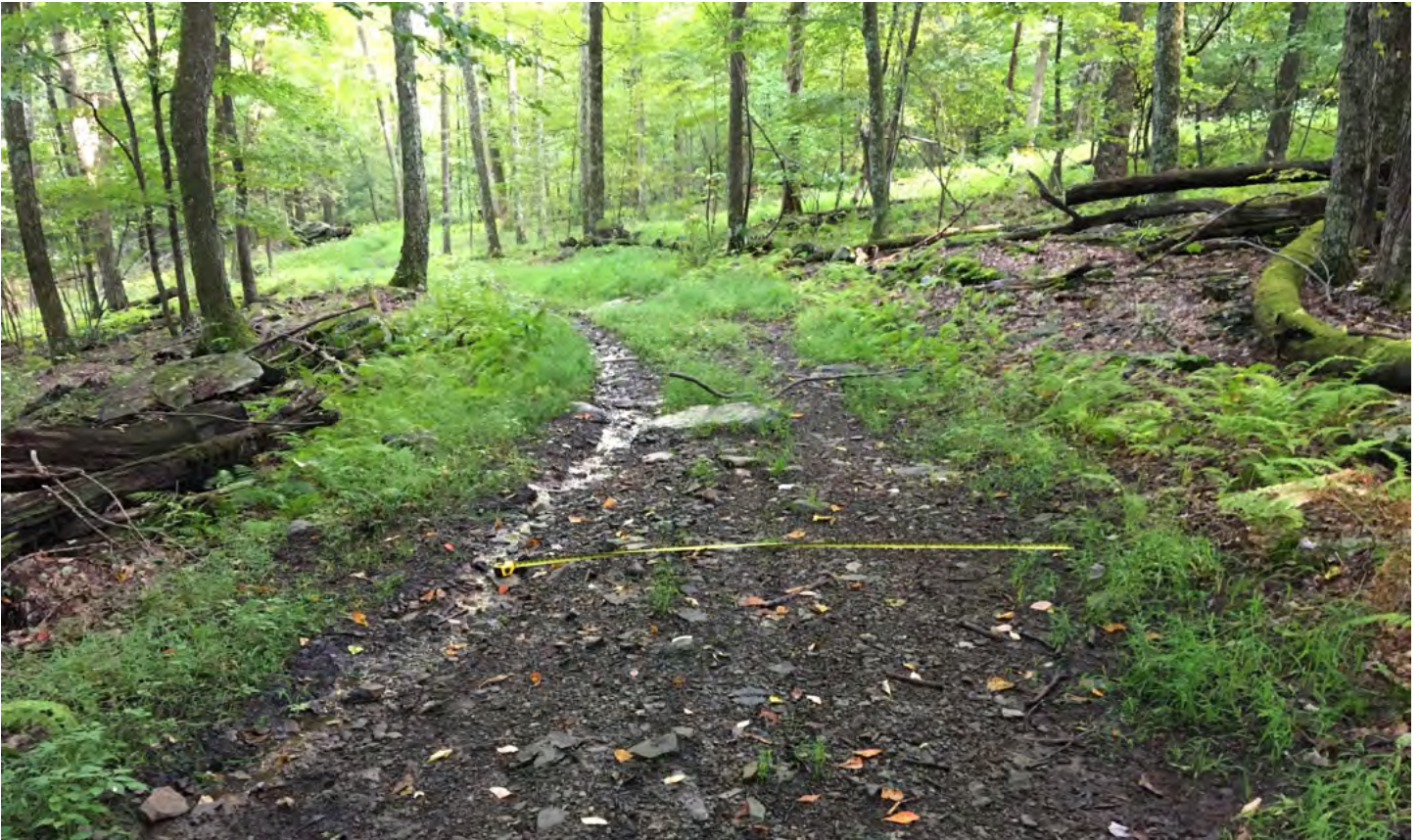
Two pictures of typical scenes from the new multi-use trail in the Vernooy Kill State Forest. The top is a 12-foot+ span as measured from the top of the benchcut to edge of disturbed area near a tree. The bottom picture shows a tape measure at a span of 8 feet in an 11-foot disturbed area.
