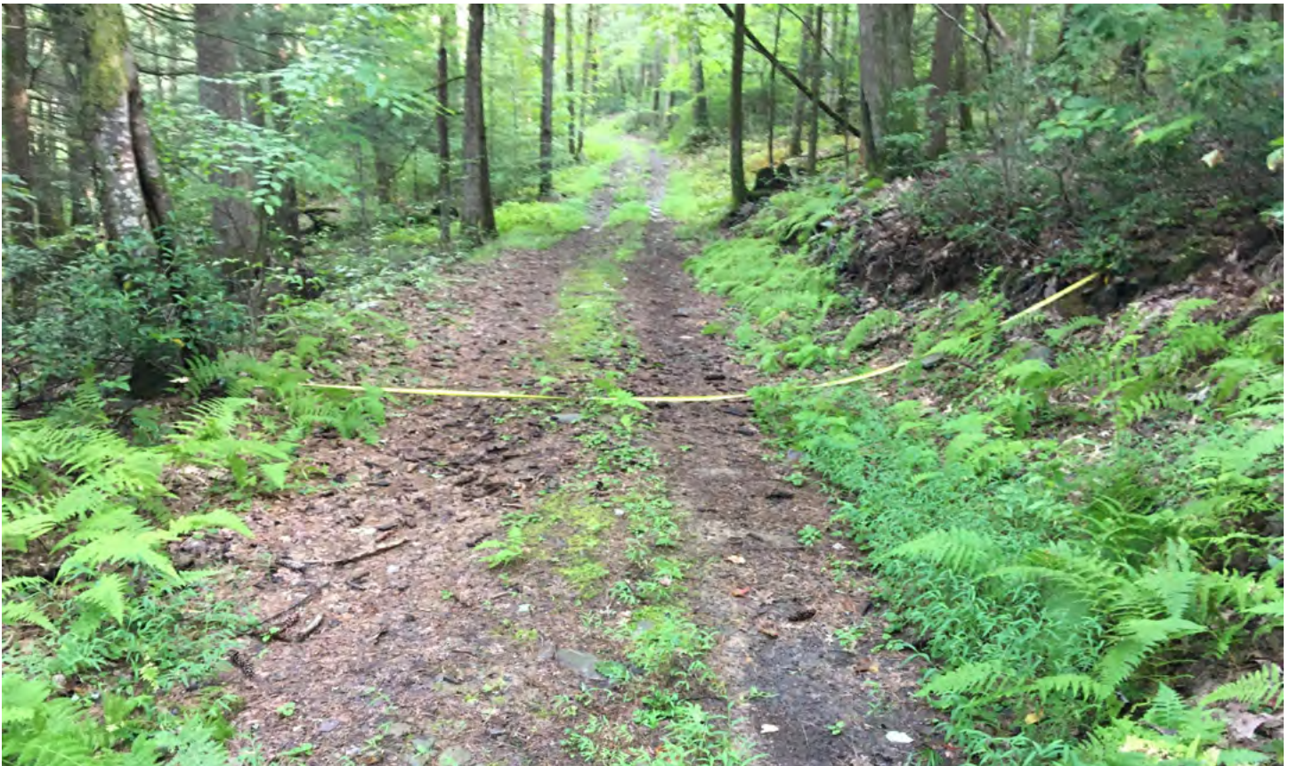
Three pictures of a benchcut from the new multi-use trail in the Vernoooy Kill State Forest, where benchcuts were widely used. The disturbed area spans 15 feet with a high bench cut on one side. This section of the trail more resembles a road than a hiking trail. This straight, flat section should have been no more than 6 feet wide.
