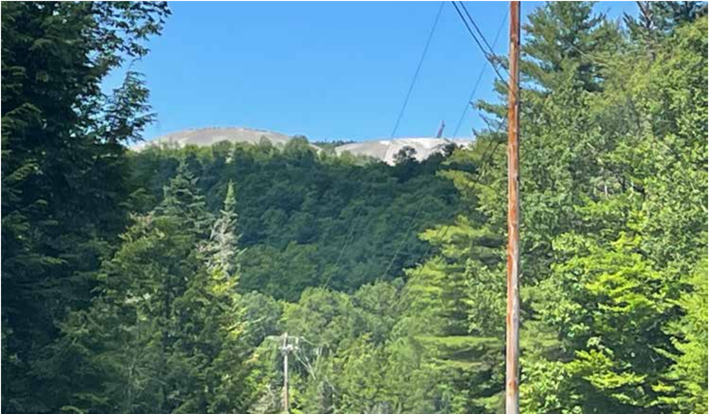
The picture shows the tailings pile as evident from County Route 78. Note the extensive exposed area. Note that visibility of industrial equipment on the right side of the pile.
