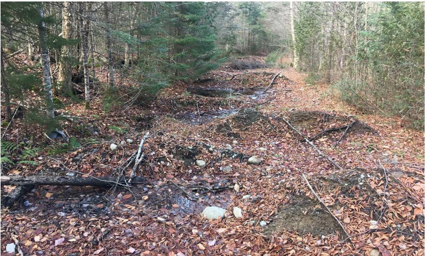
These pictures from 2021 show ecological restoration work undertaken by DEC in 2019-2020 to restore forests on abandoned logging road corridors in the MacIntyre East section of the High Peaks Wilderness. This work dismantled the road corridor and constructed a series of pits and mounds that mimic natural forest conditions.
