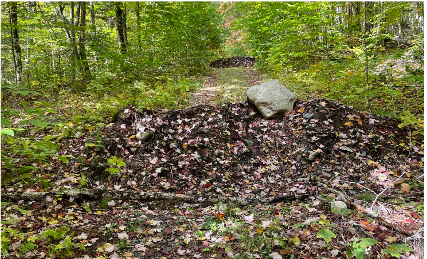
These pictures from 2022 show ecological restoration work undertaken by DEC in 2019-2020 to restore forests in abandoned logging road corridors in the MacIntyre East section of the High Peaks Wilderness. This work dismantled the road corridor and constructed a series of pits and mounds that mimic natural forest conditions.
